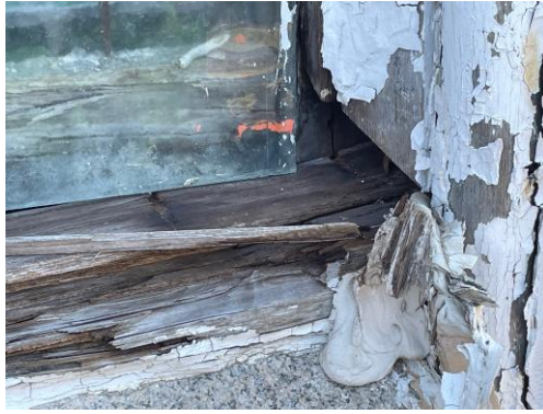
PREVIOUS DETERIORATED SILL AND BULLNOSE FRAME
